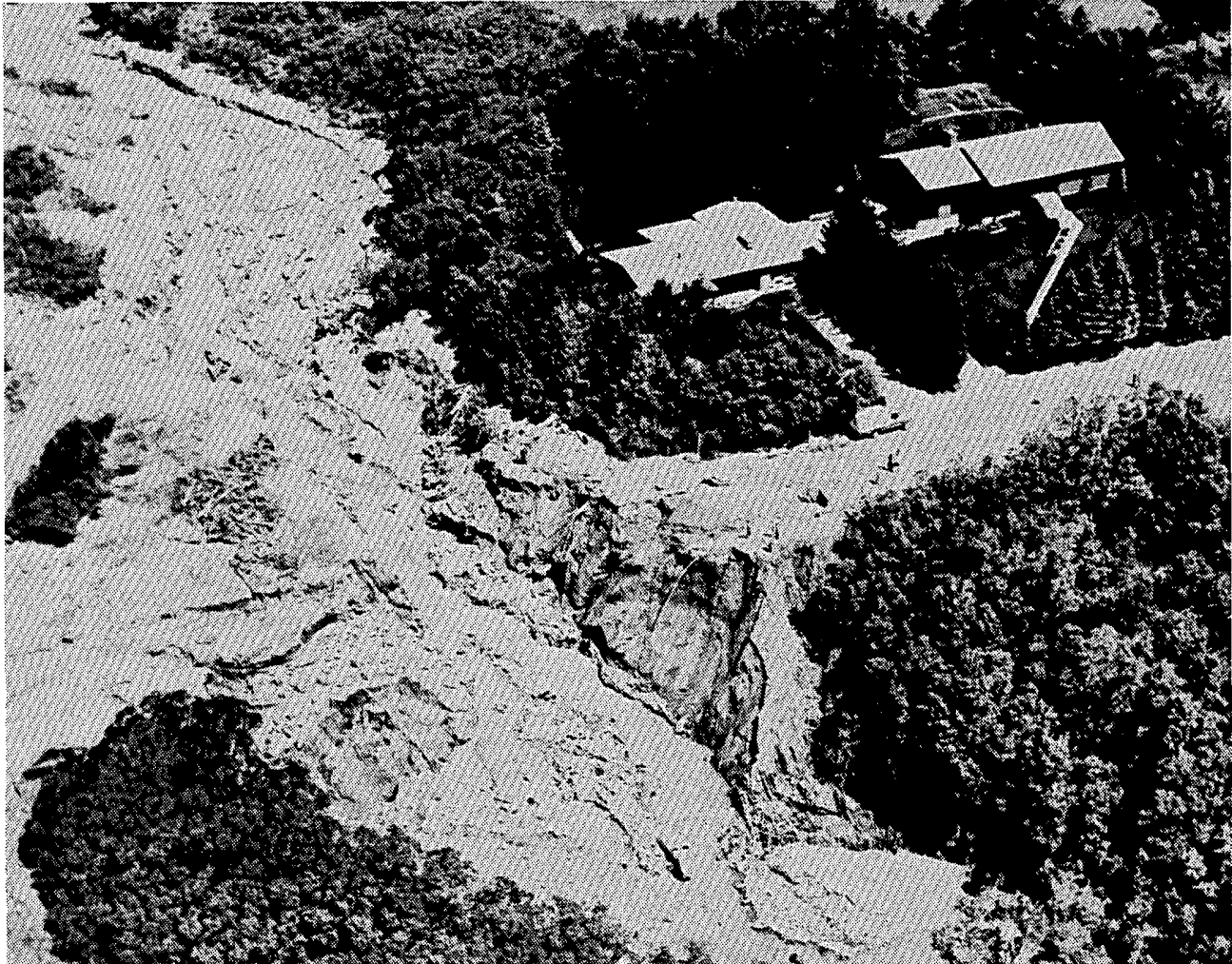
Washout of Lakeview Drive in Bountiful, Utah where it once crossed over Stone Creek. ---Photo by the Salt Lake City Tribune.
