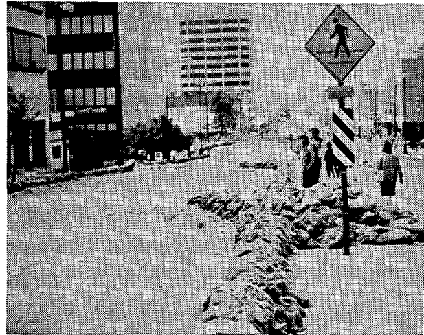
A sandbag canal on State Street in Salt Lake City, used to control excess runoff.
