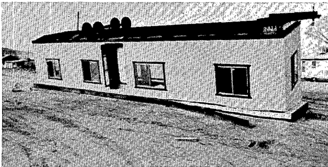
Half of a double-wide mobile home blown over.
