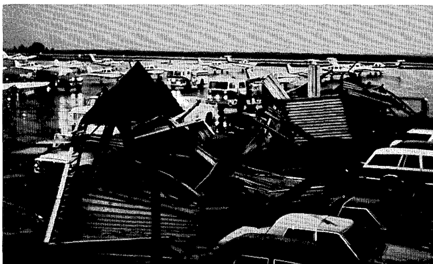
Wreckage of a hanger shown surrounded by emergency equipment shortly after the microburst. ---Photos by David Blanchard, NOAA, ERL.
