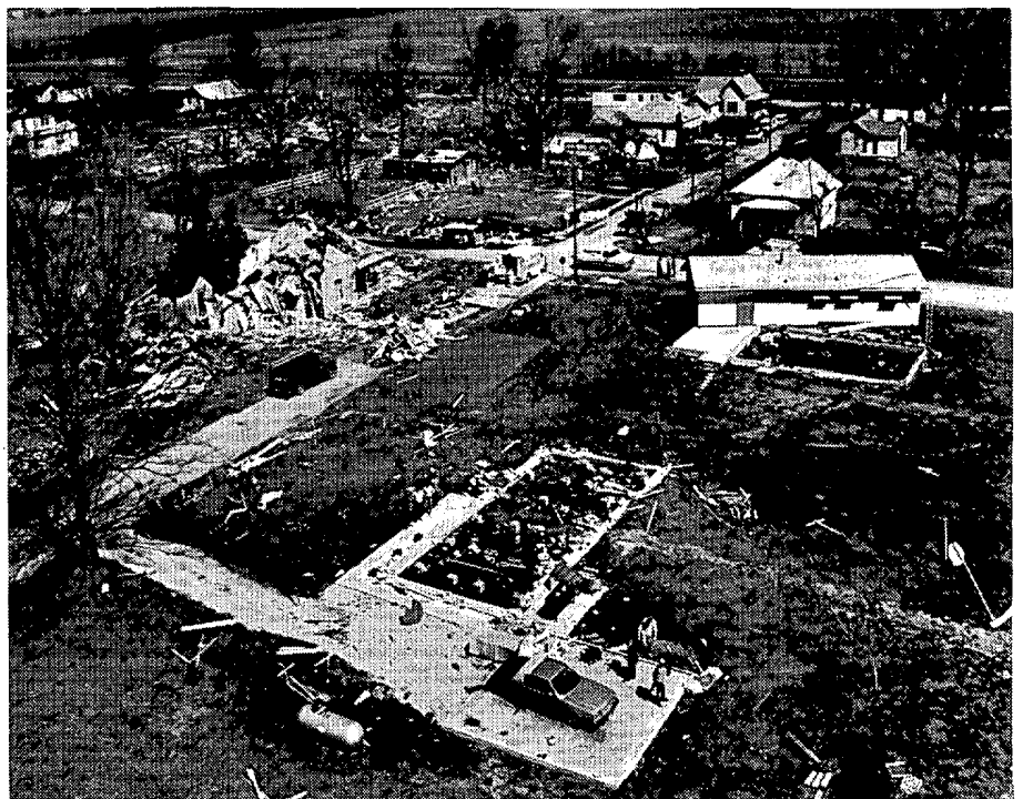
Double-wide mobile home blown from foundation (foreground) and rotated house (right center). ---Photo taken on March 31 by Paul Ockrassa, St. Louis Globe-Democrat.
