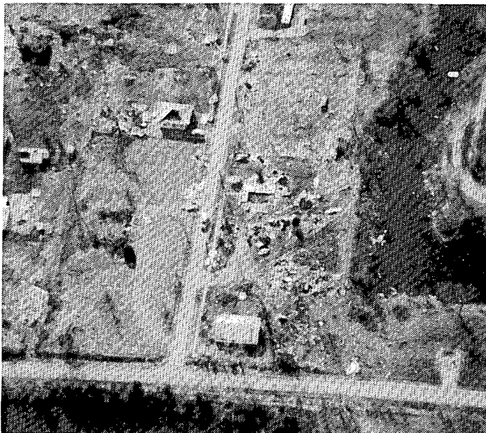
Widespread damage inside the 0.5 mile wide swath through Burgess, Mo. (UC Photo)
