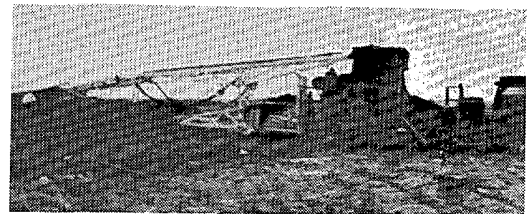
Fallen oil rig south of Winters.
