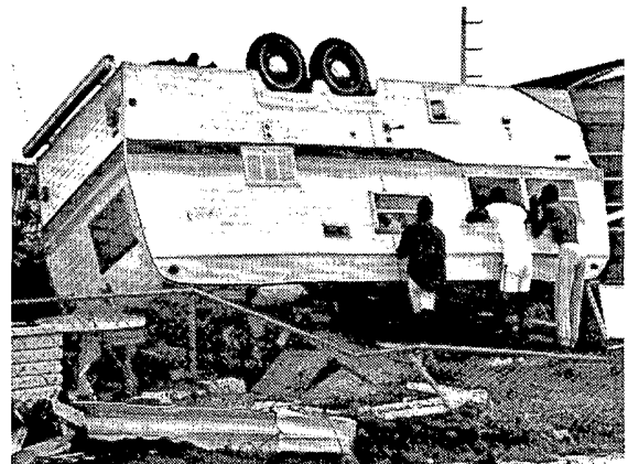
A boat trailer lifted by the tornado onto a house roof (top) and a large camper overturned at Richmond Heights. ---Photos courtesy of the Miami Herald.
