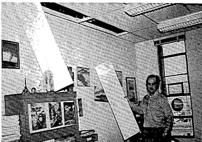
Although the exterior of the ERL office building was not damaged, some offices were disturbed by internal winds.
