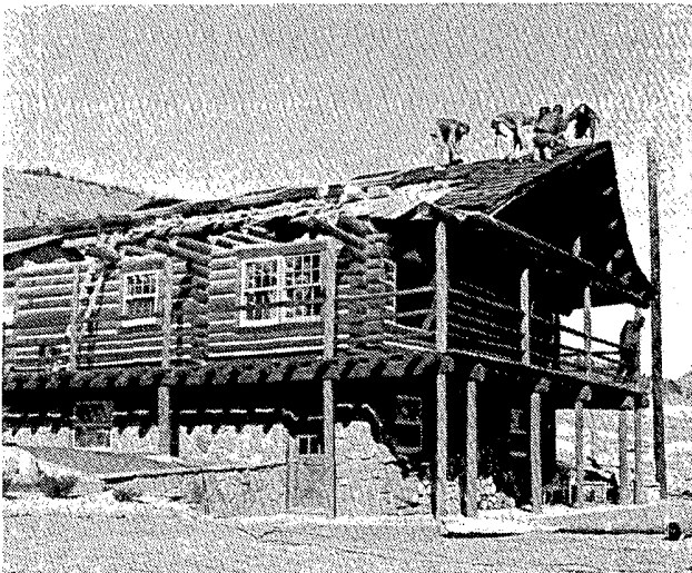
Paul Malik's house being repaired after the roof damage.
