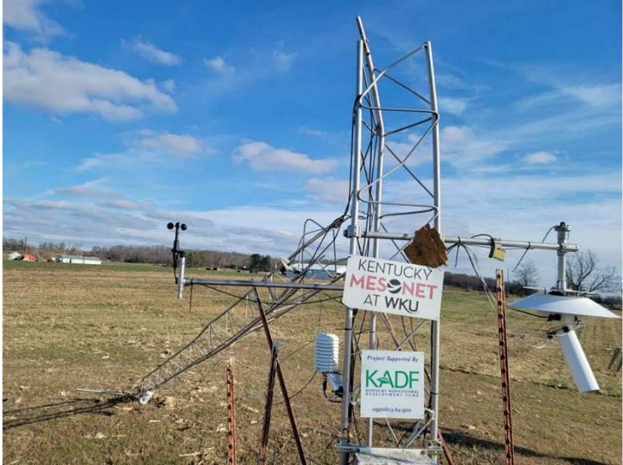
Damage to the Kentucky Mesonet's instrumentation tower in Caldwell County. While the upper part of the tower, including the anemometer mounted at 10m, failed, the lower part of the tower, including the anemometer mounted at 2m, visible on the left, remained intact and operational.
