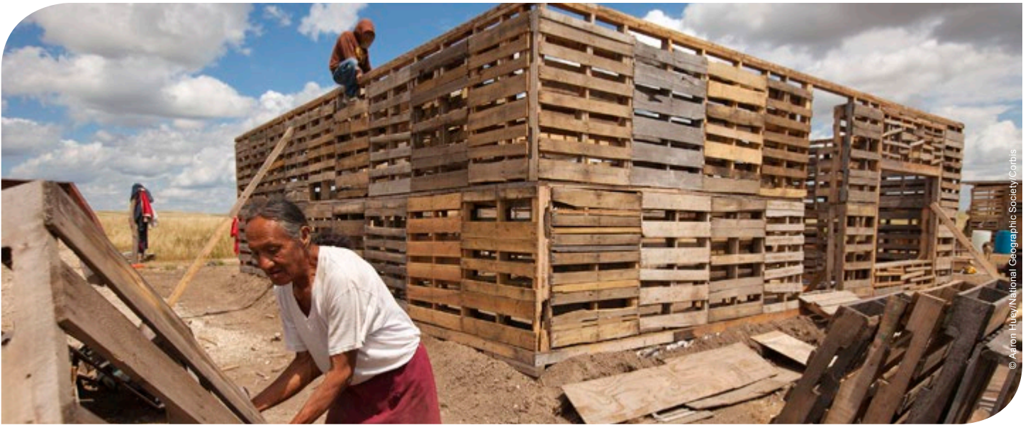
House being built on Pine Ridge Reservation
