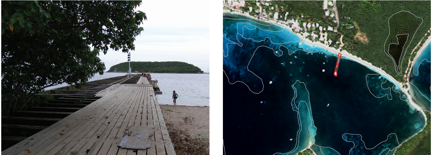
Figure 2.23. Depictions of the pier in Esperanza, an Artificial structure in Vieques. A red polygon outlines the feature on satellite imagery.
