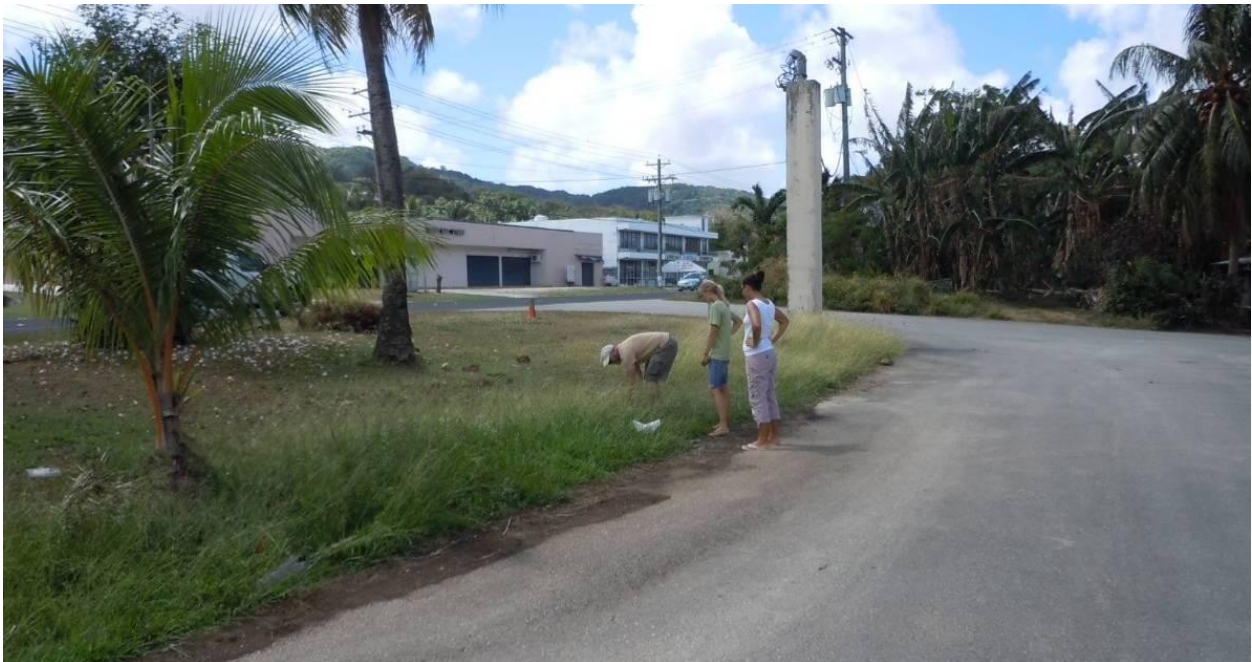
Figure 2. Rain garden location selected for installation clinic. Note evidence of ponding water and debris accumulation on edge of pavement. An existing ditch starts to the left of the small palm tree that was used as overflow from the rain garden.
