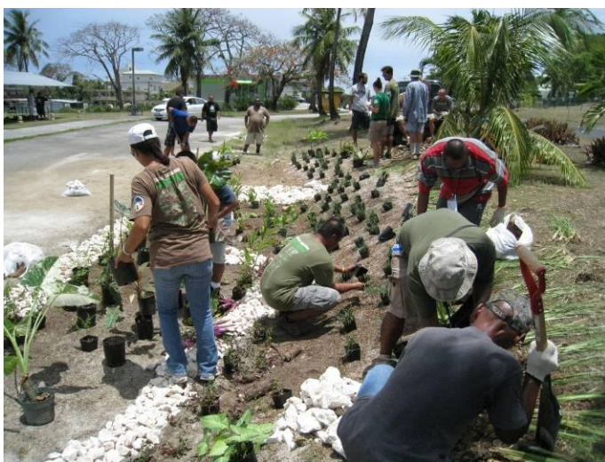
Figure 5. (From top left to bottom right) The site after major excavation the morning of the installation; amending native topsoil with coarse sand and compost; laying of stone apron; leveling of the overflow berm; placement of plants based on inundation zones; and watering of the final product.
