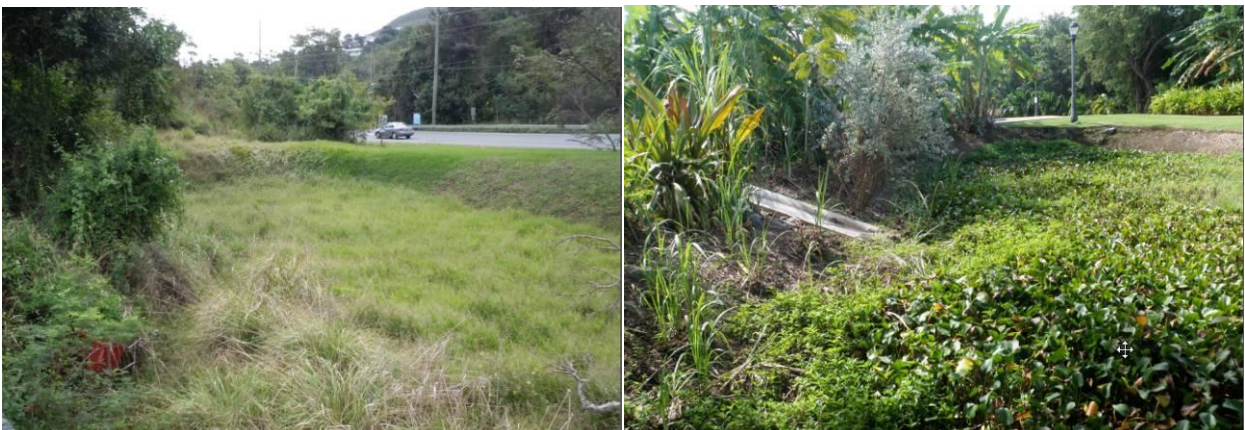
Two examples of existing stormwater management facilities are the dry detention basins at Cost-U-less and the wet basin at the Ritz Carlton.
