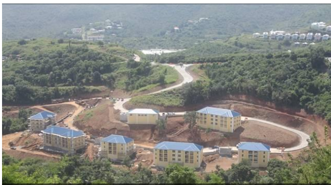
Grandview uses erosion control blankets and riprap to stabilize some slopes, but there remain acres of exposed soils and failing perimeter silt fencing that result in sedimentation downstream.
