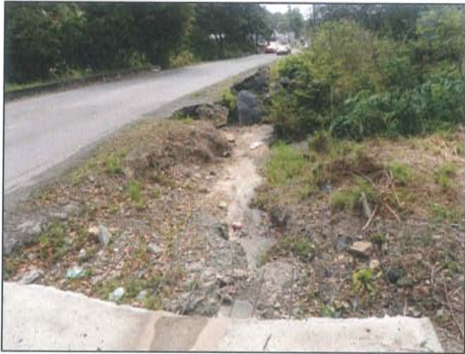
Concrete channel and scour downstream of culvert at TR-37.
