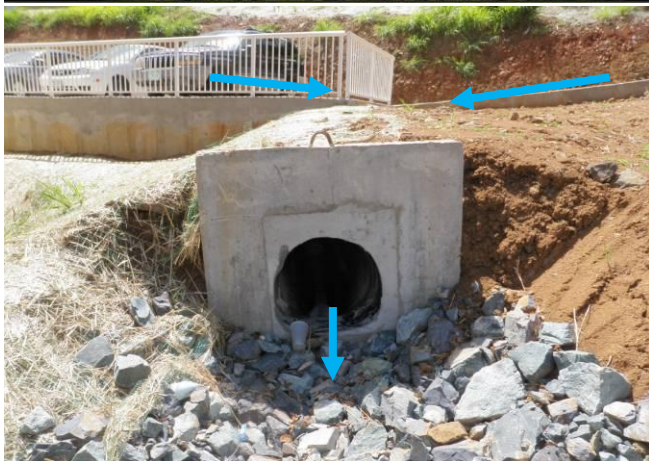
Outfalls discharge stormwater from Grandview roads and parking lots directly to the gut without any form of water quality treatment or flow detention.
