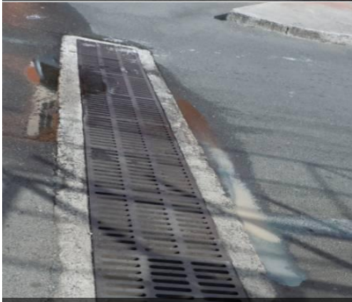
Unused cistern overflows, mop bucket waste, and dumpster juice at this site drain across the parking lot carrying pollutants into the storm drain system and discharging them downstream even when it is not
