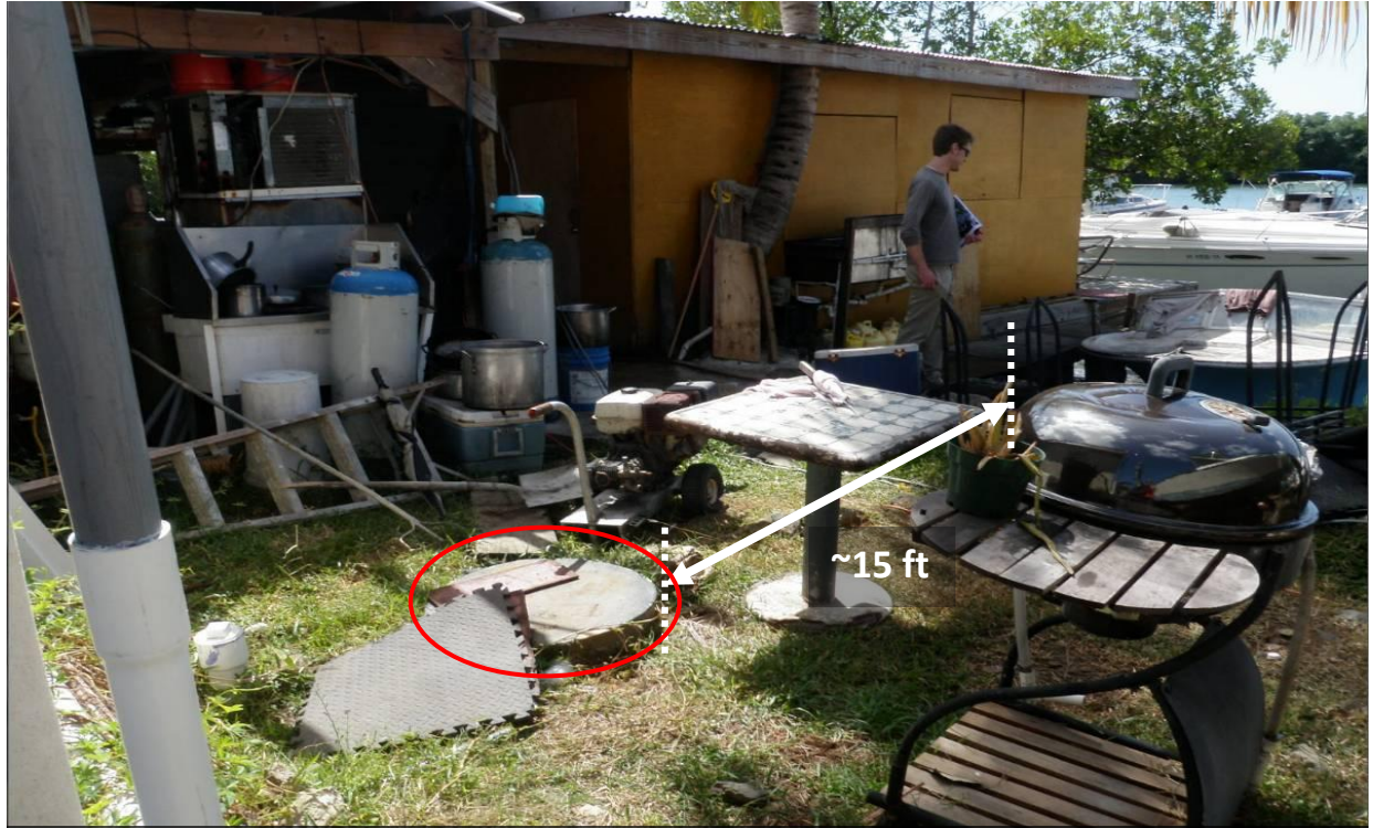
Between the restrooms and Benner Bay is the onsite wastewater system at “the Patch.” The access manhole for this OSDS is less than 15 ft from the water’s edge, leaving little distance for groundwater
