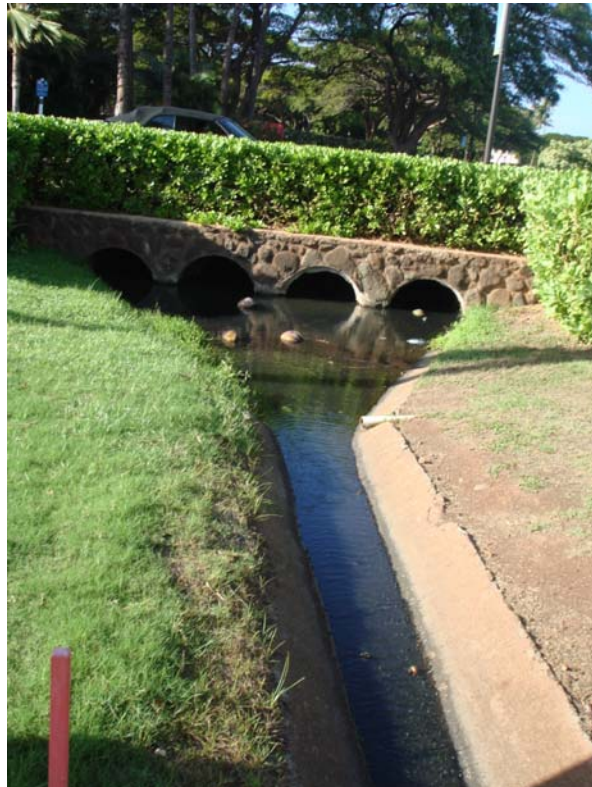
MWU3: Drainage Ditch, Dry Weather Period Flow Drains into Golf Course Ponds
