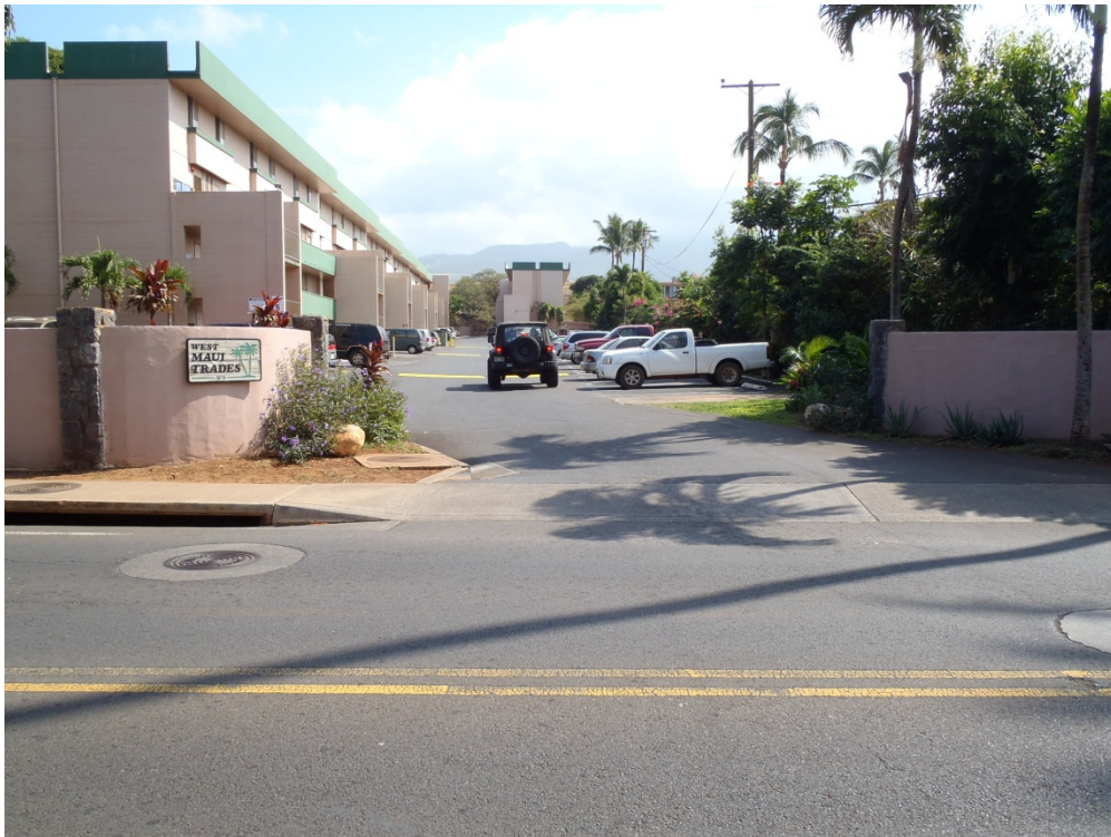
HU2: Lower Honoapiʻilani Road, Typical Parking Lot Sloped to Road Fitted with Drainage Inlets
