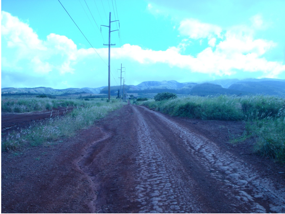
3 4 WA14: Exposed Heavily Eroding Road in Upper Elevations of Agricultural District, Running Mauka to 5 Makai (No BMPs Present)
