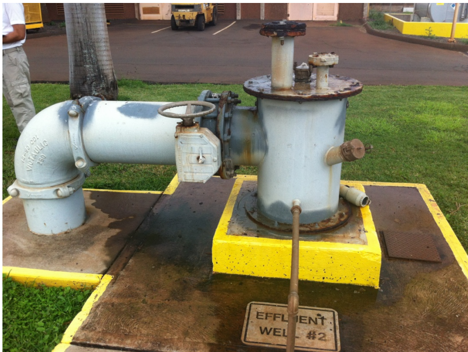
HU4: Lahaina Wastewater Reclamation Facility, Injection Well # 2
