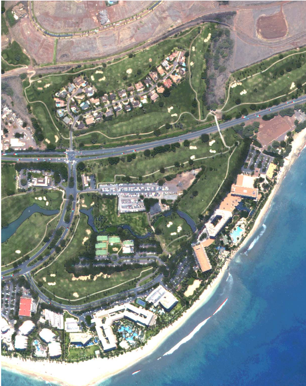
MWU5: Air View, South Half Resort Area
