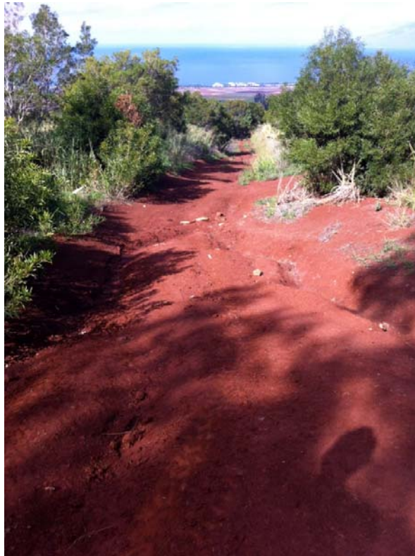
3 4 WA14: Exposed Heavily Eroding Road in Upper Elevations of Agricultural District, Running Mauka to 5 Makai (No BMPs Present)
