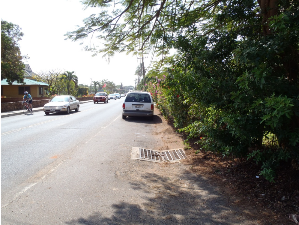
HU2: Lower Honoapiʻilani Road, Typical Parking Lot Sloped to Road Fitted with Drainage Inlets
