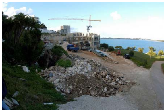
Excavation for new resort and golf course
