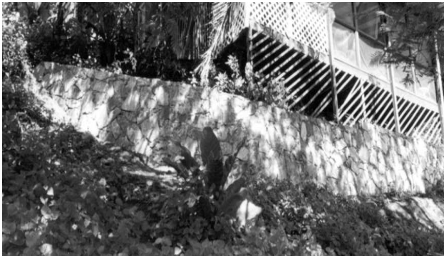
Photograph by: Dale Morton, UVI-CES
