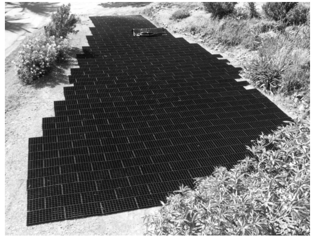
Photograph by: Dale Morton, UVI-CES
