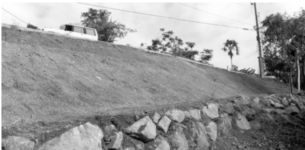
Photograph by: Dale Morton, UVI-CES
