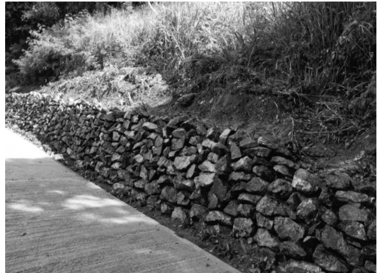
Photograph by: Dale Morton, UVI-CES
