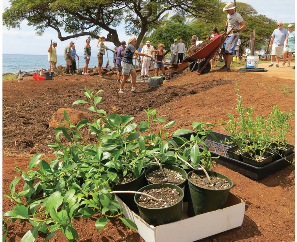
Volunteers install a rain garden at Wahikuli Wayside Park.
