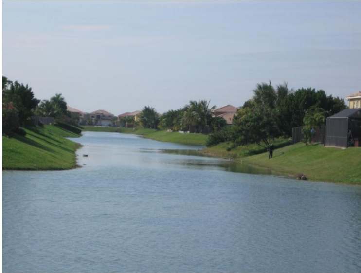
Figure 14. This pond, in Miami-Dade County does not incorporate some features that would improve its performance, such as shallow side slopes, an “aquatic bench” that promotes growth of wetland vegetation and irregular geometry. Photo Source: CWP.
