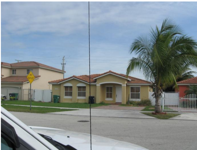
Figure 12. A combination of local codes, such as off-site parking requirements, street widths, and sidewalk requirements work together to increase impervious cover in this residential development.
