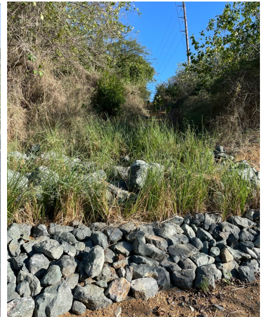
Example of a hybrid road closure technique in Culebra used to close roads.
