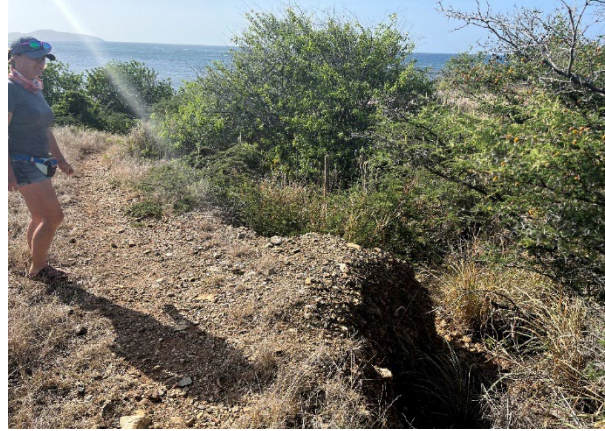
Existing conditions. West Trail. 2024.
