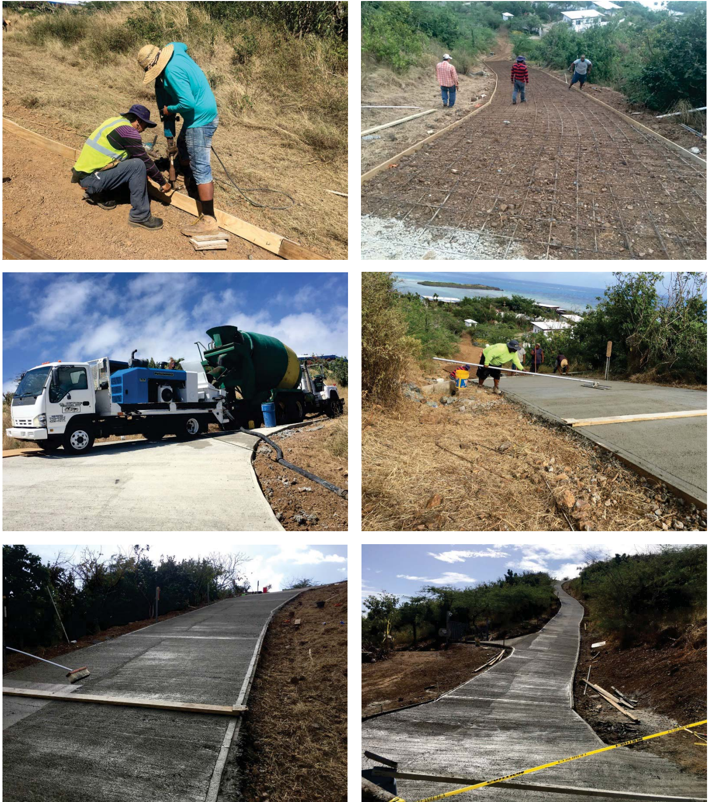
Figure 16. Rebar installation and concrete pouring.
