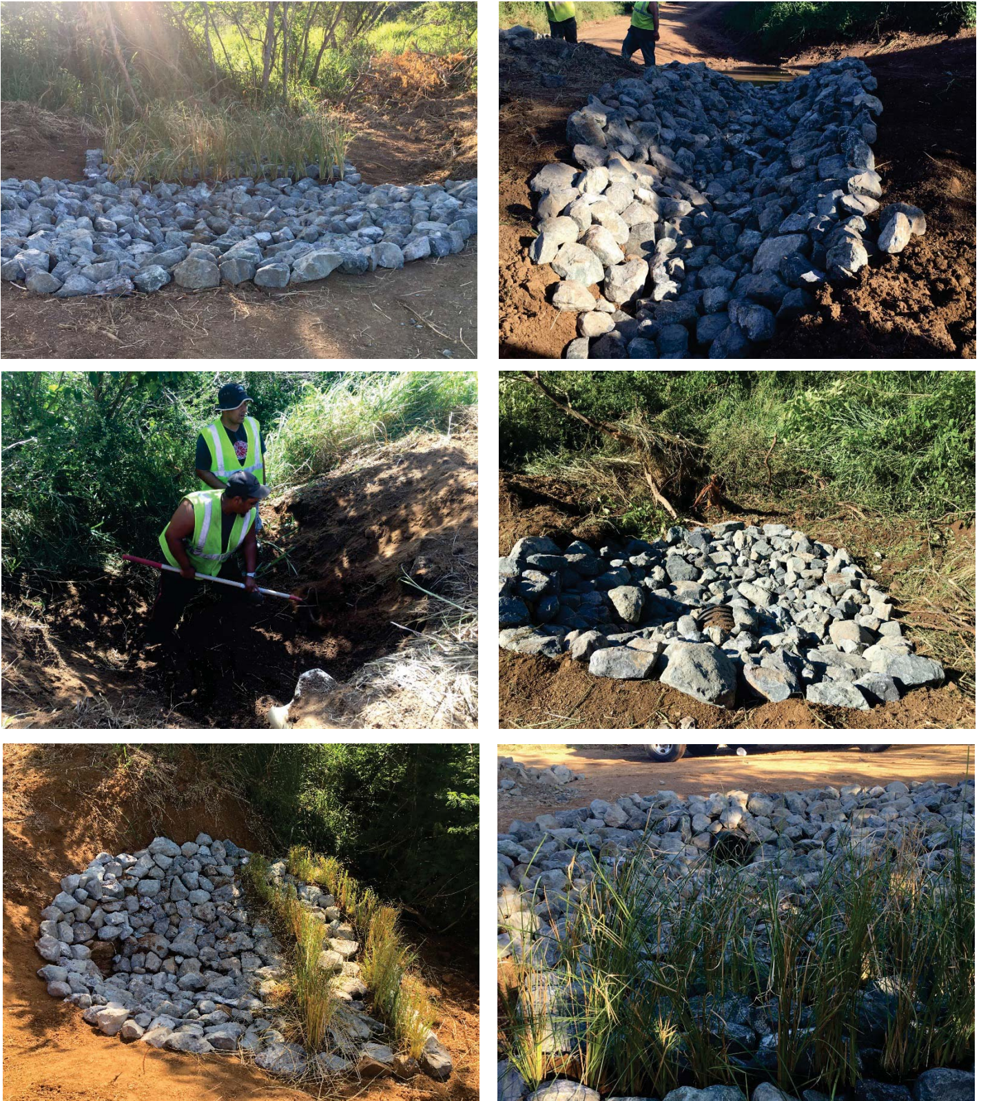
Figure 8. Installation of rip-rap and Vetiver on the outfalls of crossing pipes.
