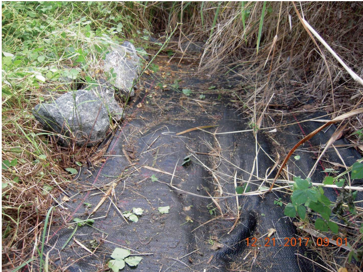
Figure 30: Sediment apron at a check dam in Punta Aloe
