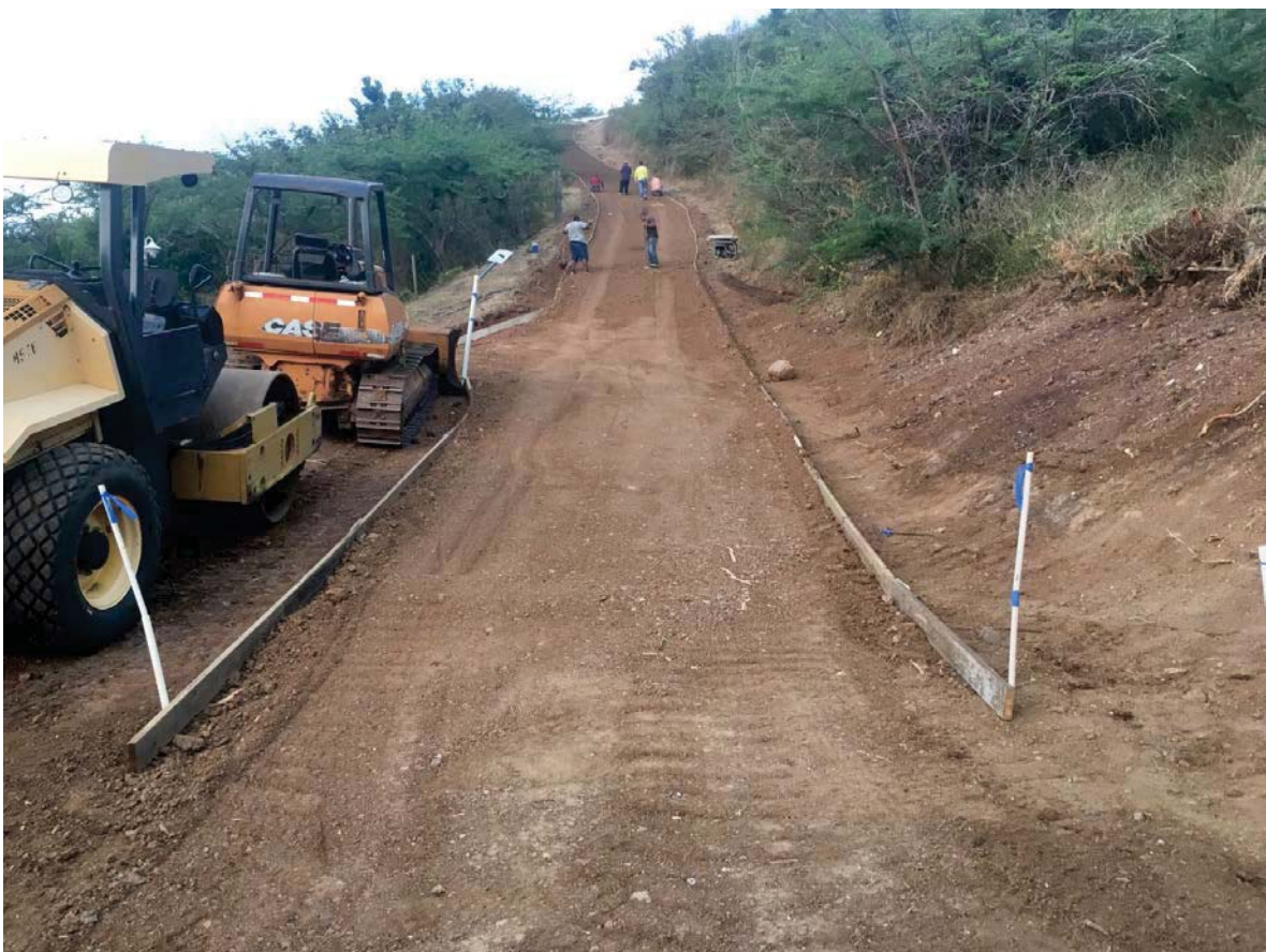
Figure 15. Molding preparation for concrete paving.
