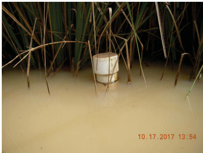
Figure 27: Water level recorder installed at the detention pond in Punta Aloe
