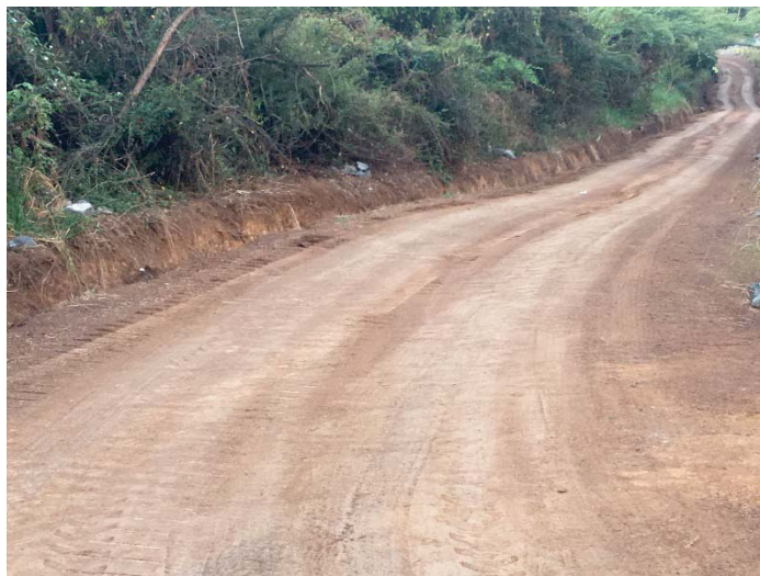
Figure 3. Regrading and compaction process during dirt road stabilization.
