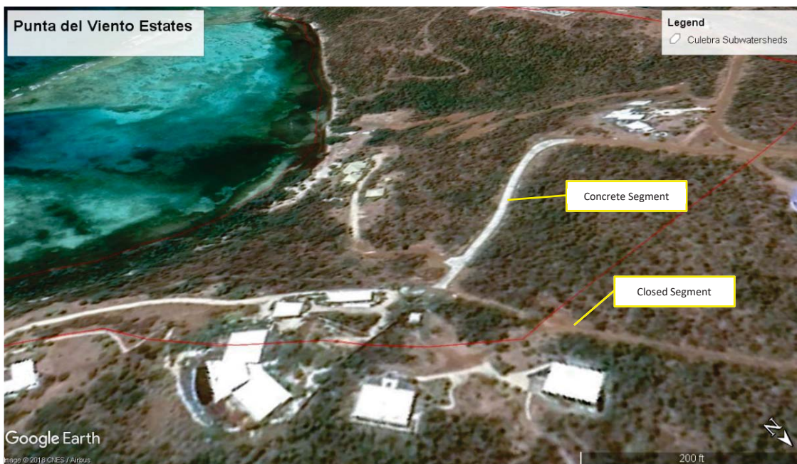
Figure 13. Aerial image of the project site area showing the concrete pavement and part of the closed dirt road segment.
