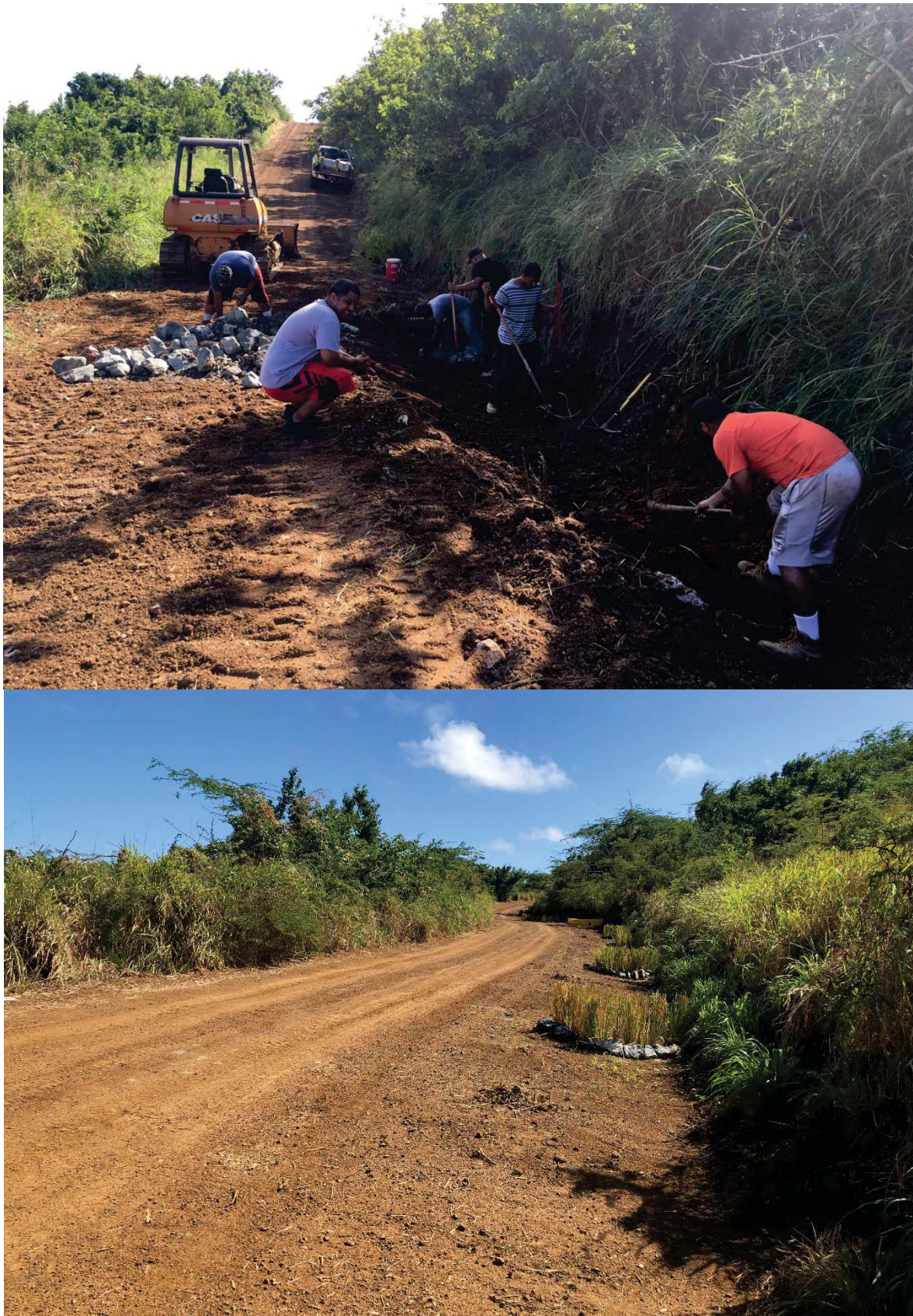
Figure 1. Construction process of installing check dams.
