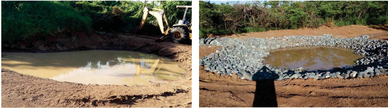
Figure 12. Example of a rain event captured by the sediment traps during project implementation.
