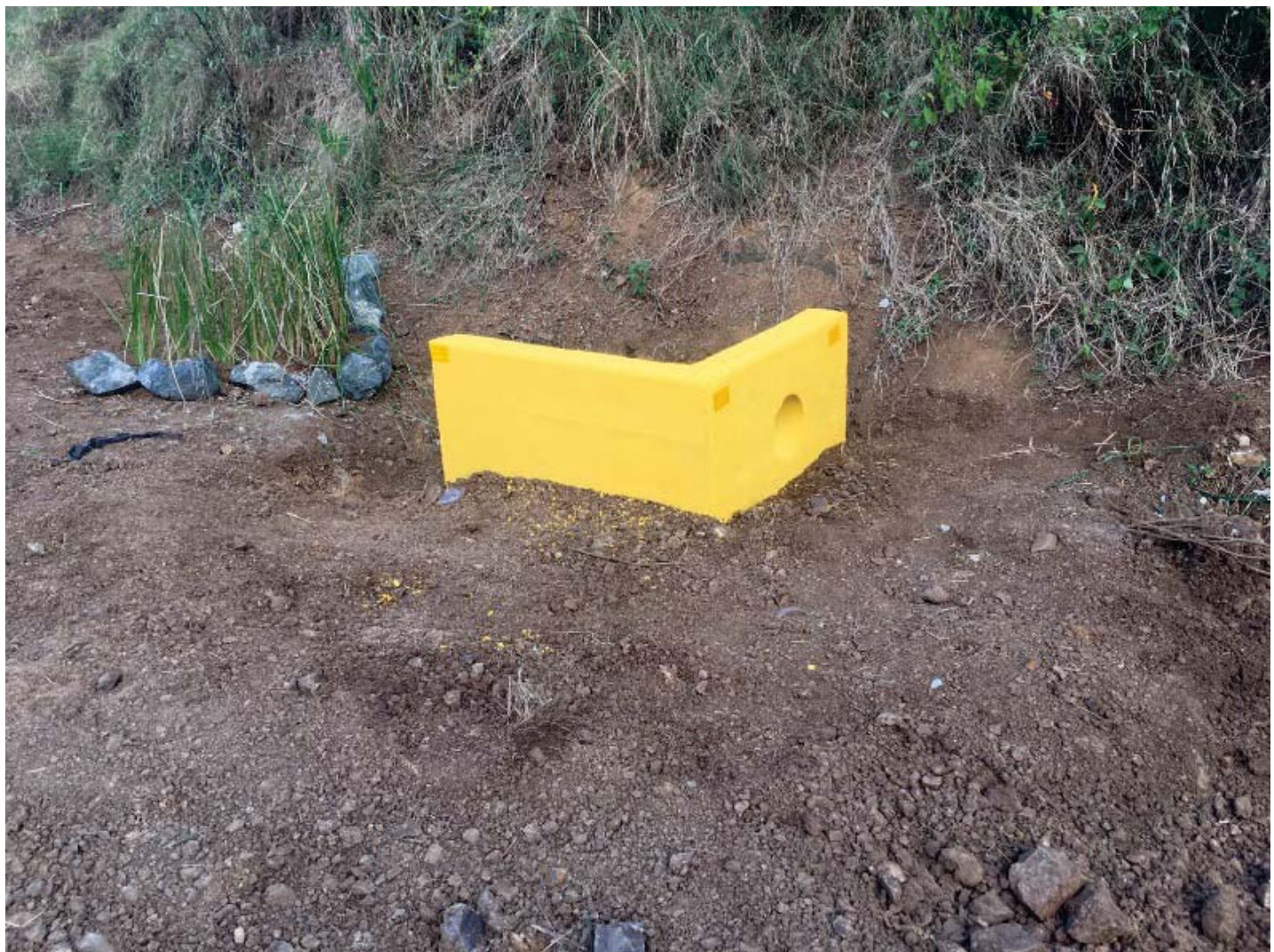
Figure 7. Construction process of installing concrete catchments for the crossing pipes.
