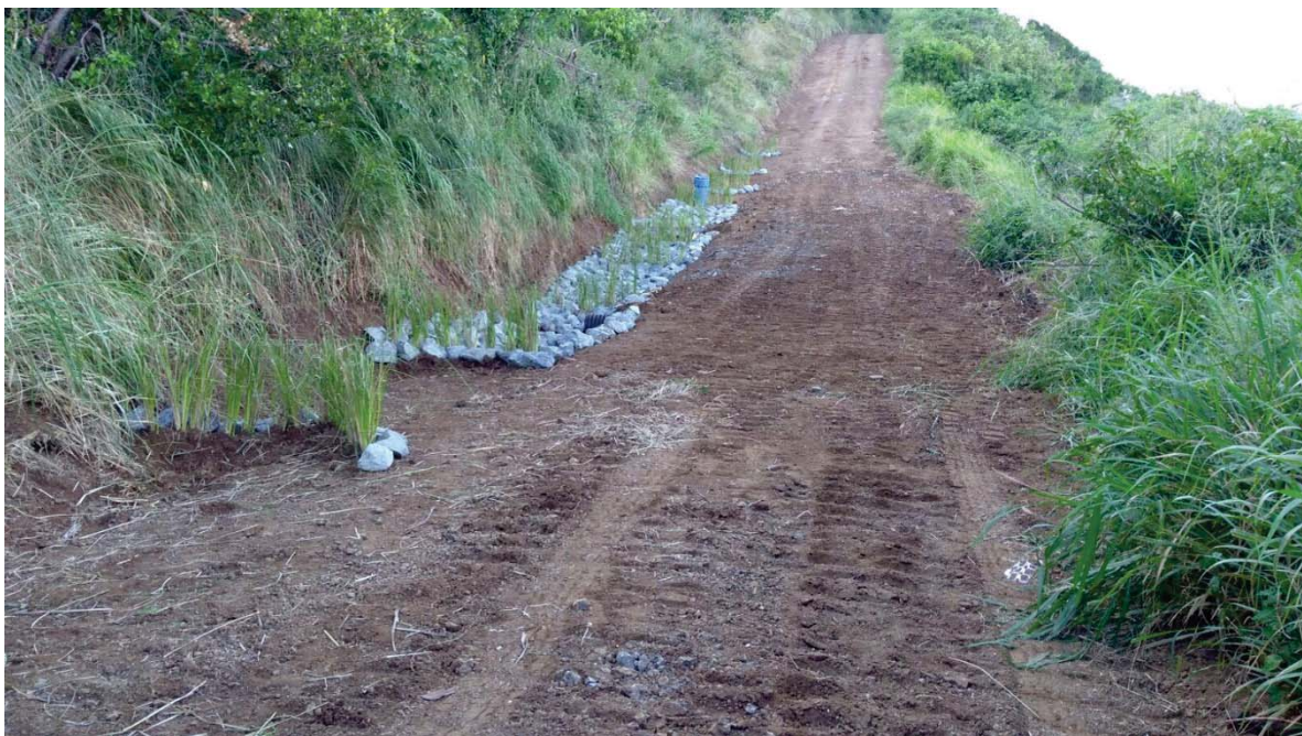
Figure 9. Installation of rip-rap terraces.
