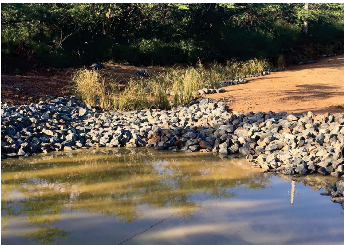
Figure 10. Example of one of the sediment traps constructed.
