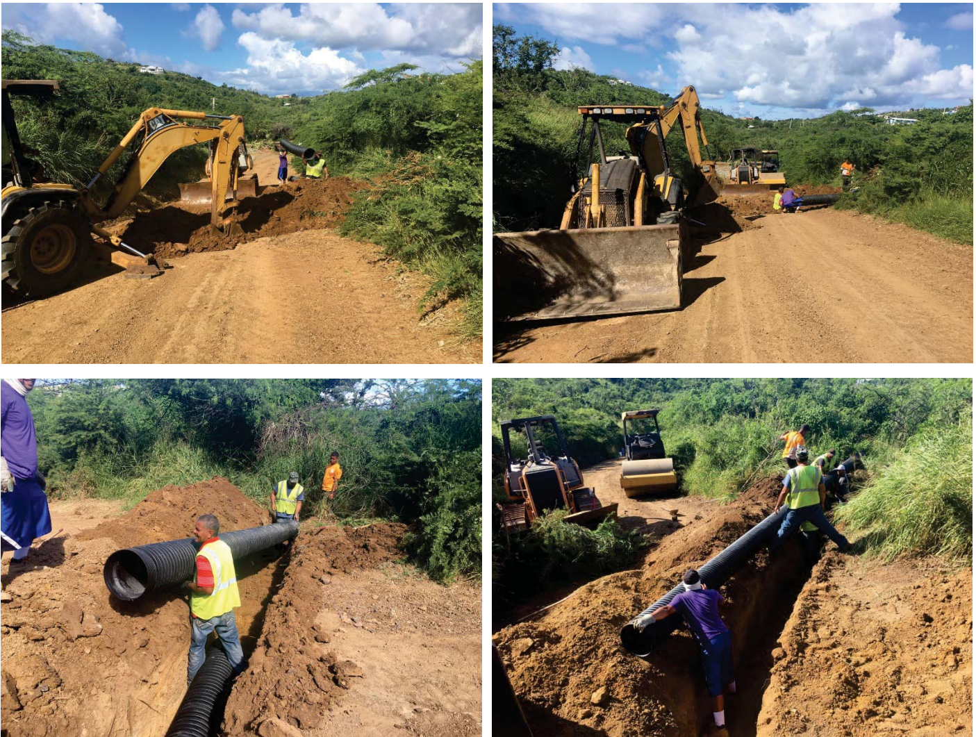
Figure 5. Process of installation of crossing pipes.
