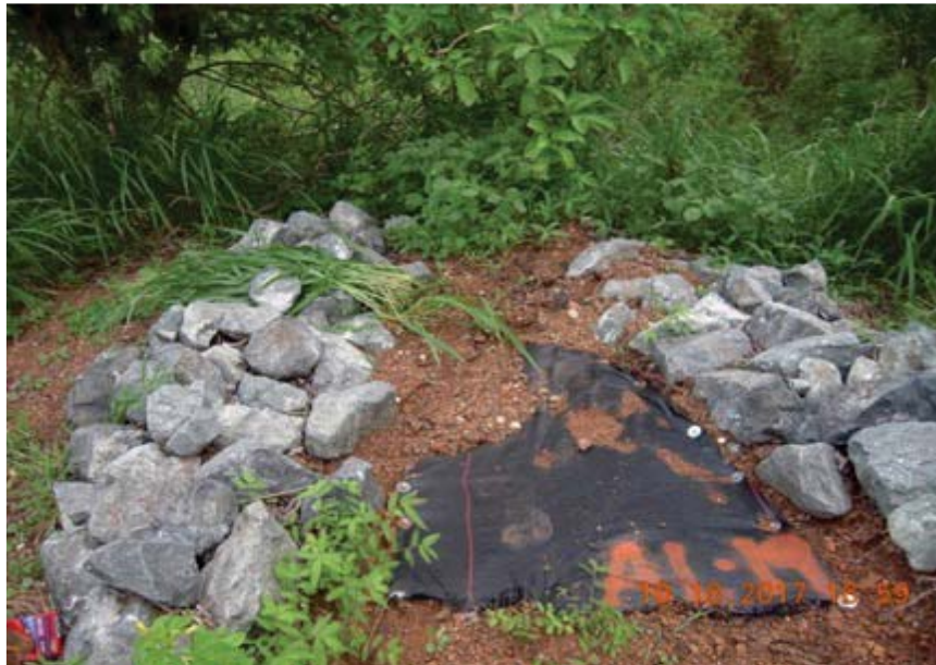
Figure 34: Trap 19, note how the sediment goes over the energy dissipating
