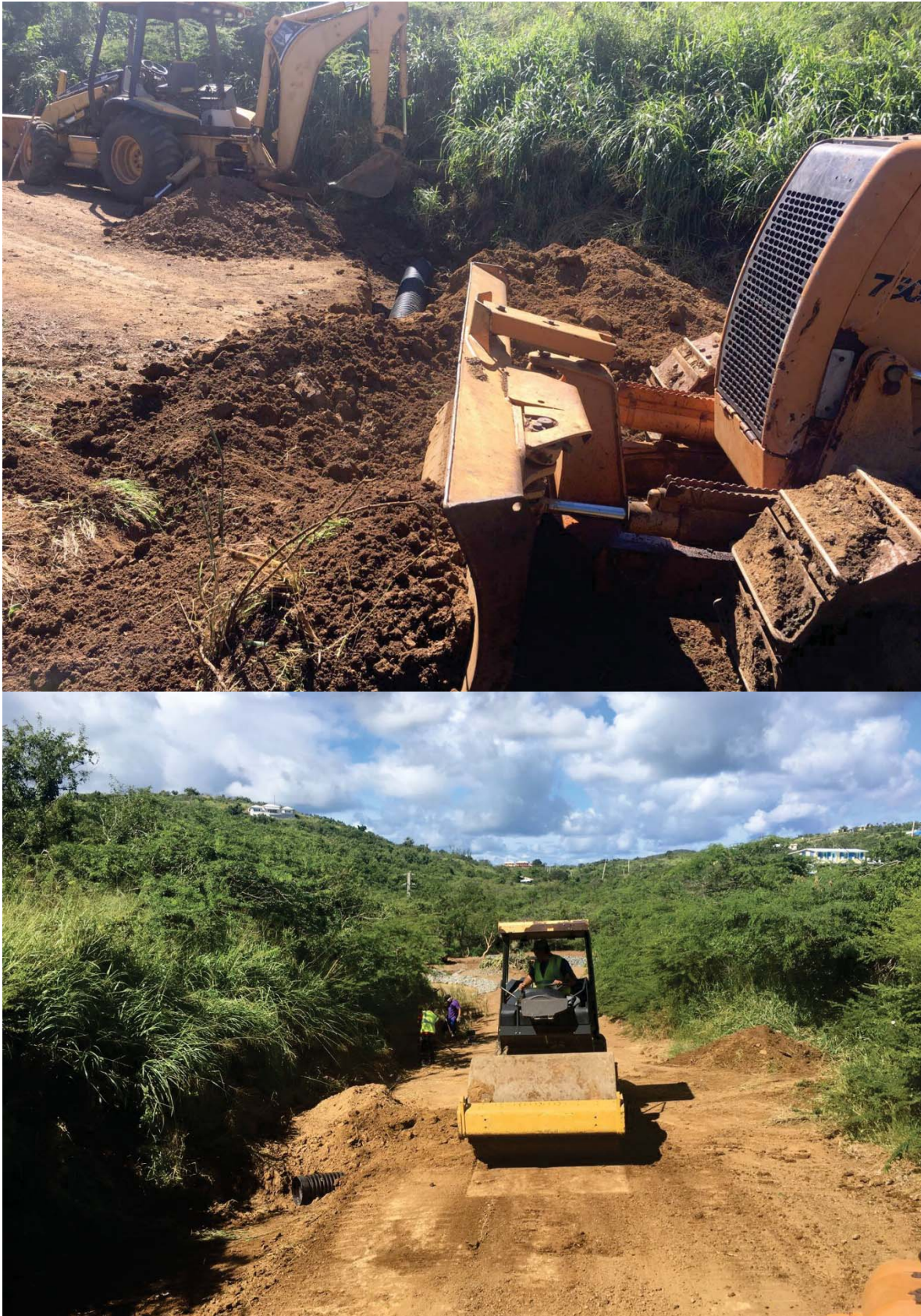
Figure 6. Regrading and compaction of road after installation of crossing pipes.
