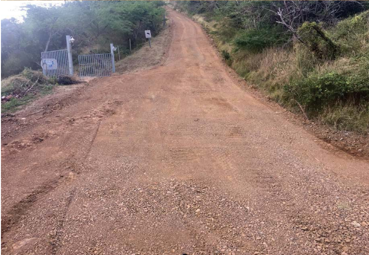
Figure 14. Regrading and compaction process prior to concrete paving.
