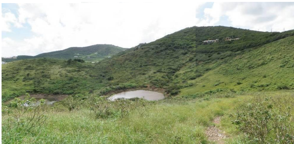
Figure 5.2. Skov farm ponds. The pond on the left is leaking, the one on the right is receiving sediment from hillside erosion.
