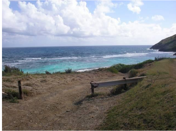
Figure 5.5. Open guardrail off East End Rd.
