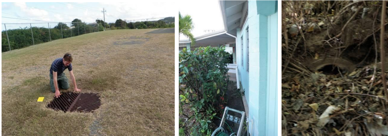
Figure 3.12. Drain inlet in lower parking lot (left); downspout to existing flowerbed that could be converted to a rain garden or collected for irrigation (middle); almost completely blocked culvert (right).
